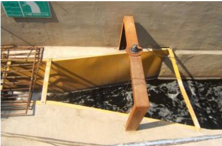
Figure 4.3.3 Parshall flume
