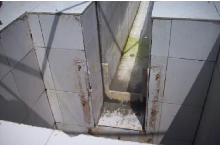
Figure 4.3.2 Rectangular Weir
